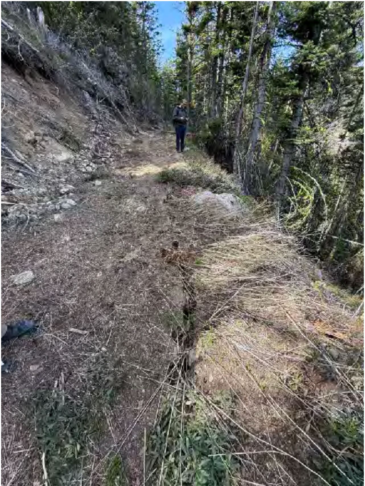
Part of the roadbed of the illegal road is cracking and sloughing downslope. One of many ongoing erosion features that are actively impacting forest health, and in some locations, within the riparian buffer of Squilchuck Creek.
